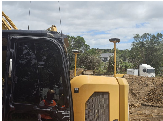
Cat excavator on site with RS4 base visible in background
