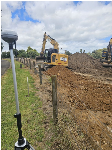
RS4 base station (foreground) with Cat excavator at work on site
