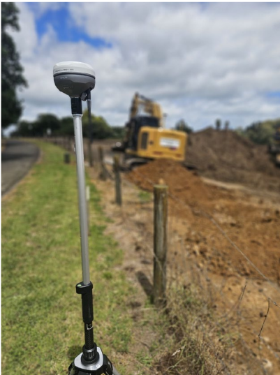
RS4 on site at a residential subdivision
